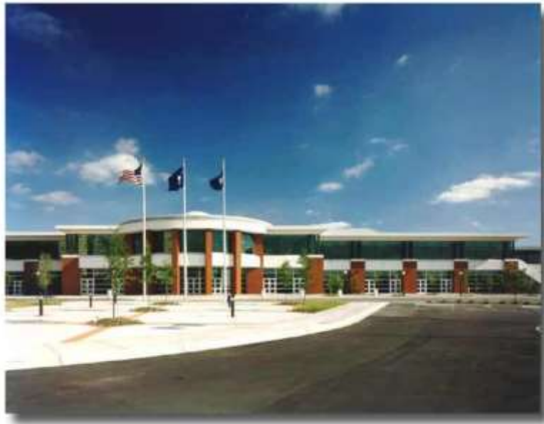
Figure 10. North Charleston Convention Center is a great venue to display and demo the MHRS.
